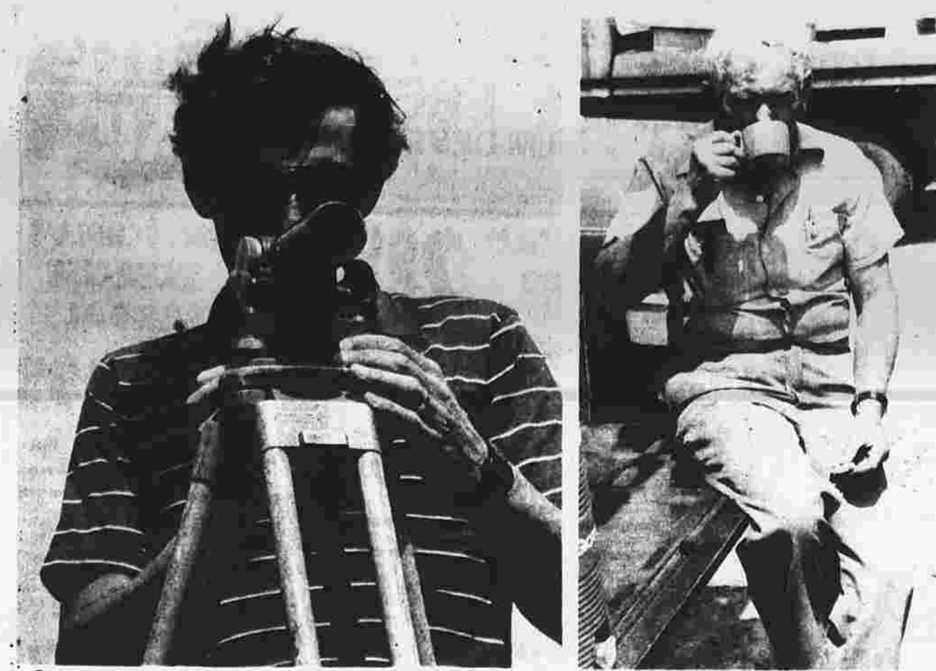
Surveyor Richard Atwood of the Brunali Construction Co. checks out the angle of a bridge abutment over Buckland Street.
